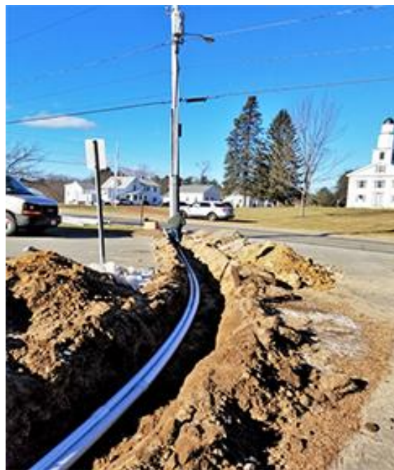
New Conduit Burial from Cooleyville Road to our hut behind Town Hall
