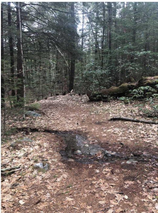
Photo 16. Streamlet crosses trail. Drain working well but monitor annually.
