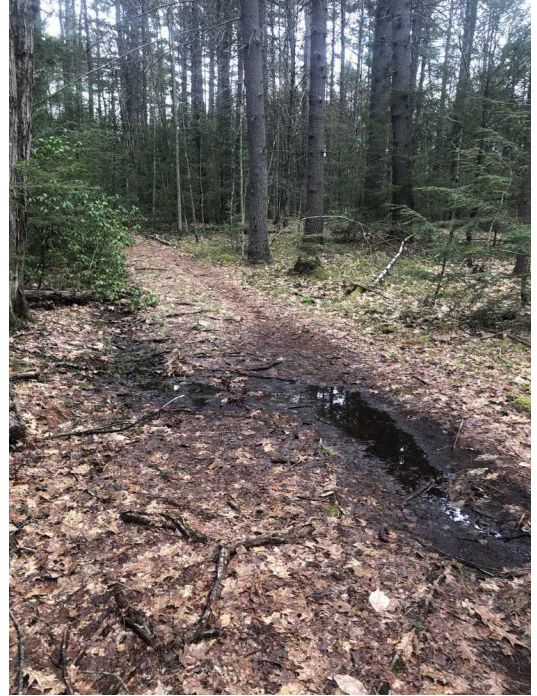
Photo 15. Stream let forming puddle - dig drain to shed water off the trail.
