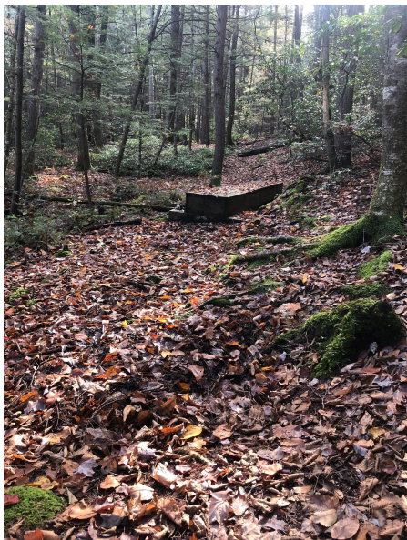
Photo 3. Mudhole forming near bridge. 10' bog bridge recommended.
