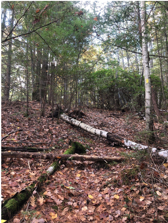
Photo 7. Steep slope and two blowdowns on trail. Remove blowdowns, monitor slope for erosion, and Consider hardening (gravel, rock steps)
