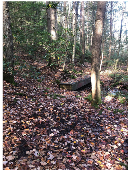
Photo 4. Mudhole forming near bridge. 10' bog bridge recommended.
