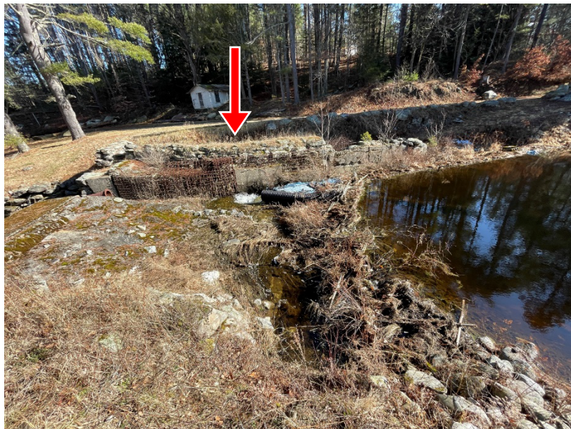
Photo 4. Overview of the dam spillway and beaver dam from the left spillway abutment; note location of void space behind the right dam wall
