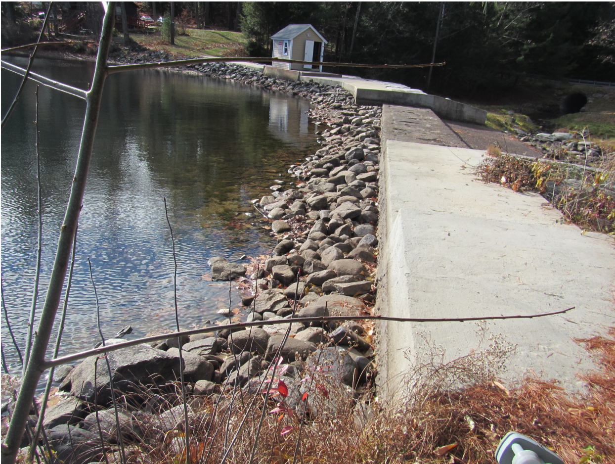
Lake Wyola Dam - November 22, 2016
