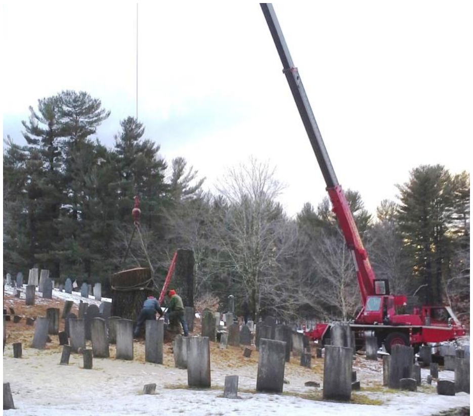
Workers from Cotton Tree Service prepare to hoist the remaining stump of a white pine from the earth in January. Seven white pines in West Cemetery were removed to prevent further damage to historic grave stones caused by heavy branches dropping from old and ailing trees. Town Meeting approved the use of Community Preservation Act funds for this project in 2015.
