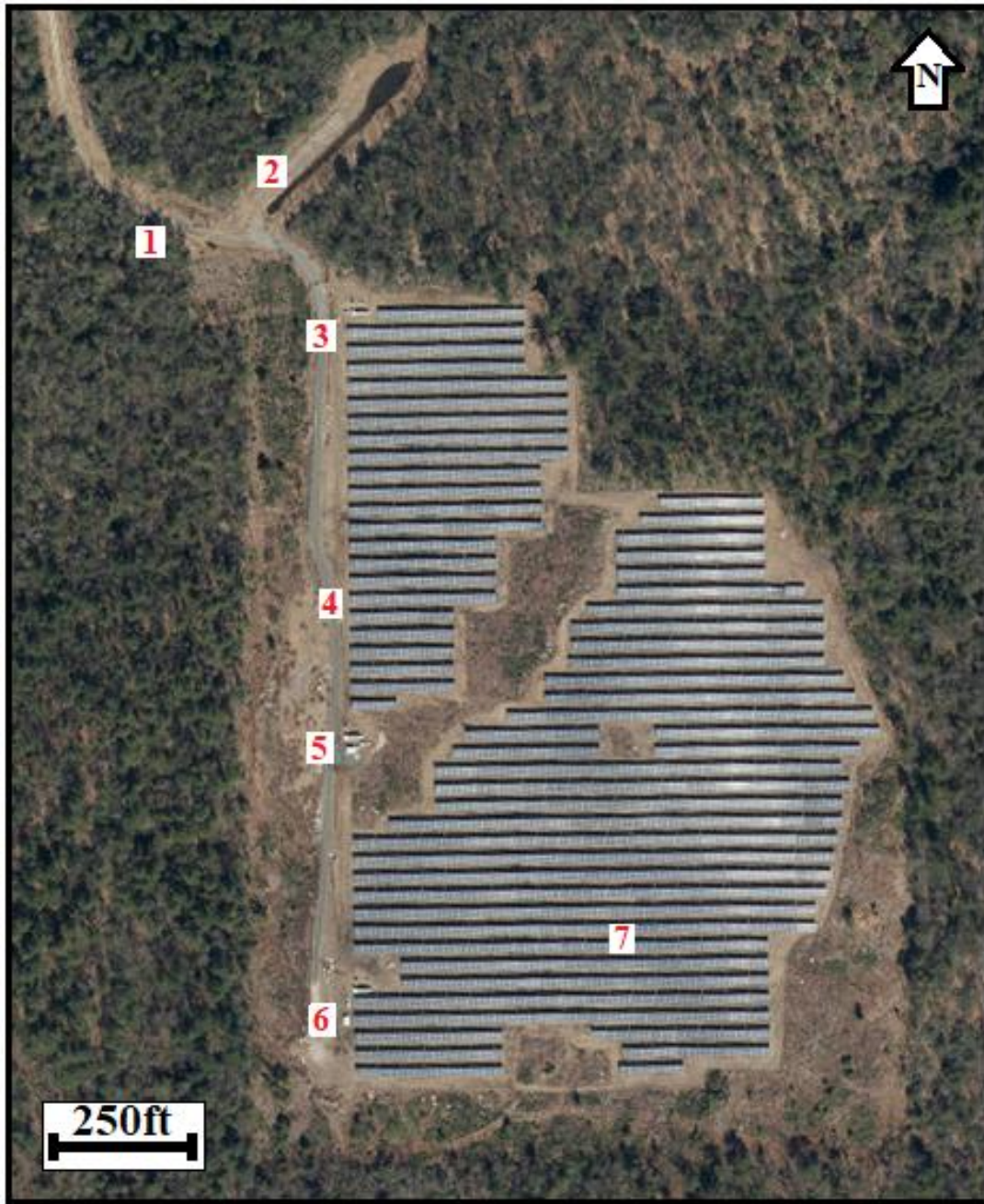
Figure 2. Aerial photograph of the Nextera Energy, Inc Shutesbury solar facility. Numbers in red correspond to the locations and photographs discussed below (MassGIS 2023 imagery, accessed August 13, 2024).
